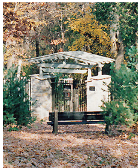
The new front gate to Eloise Butler shown in the Fall of 1992 after the upper arbor was installed but before the inscription. Photo ©G D Bebeau
