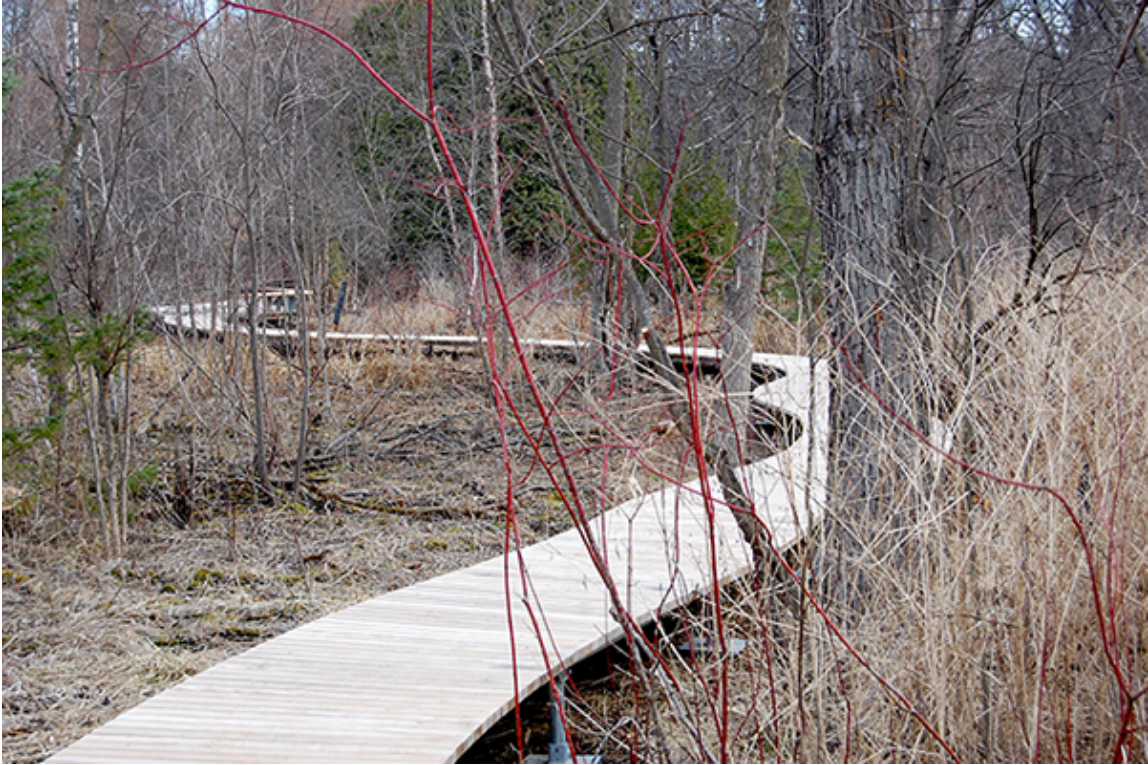
Below: The curving sections of the new phase. Photo G D Bebeau
